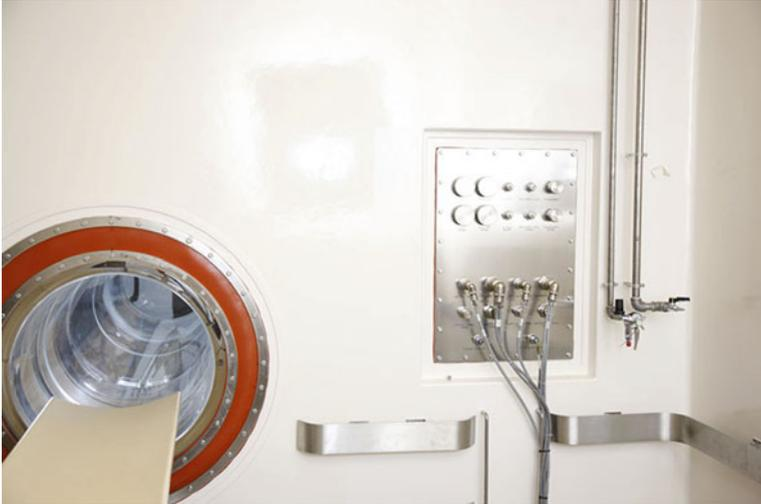
**Fig. 10.2** Airtight patch panel through which electrical signals are sent to electronic components on the cold side of the barrier wall. This eliminates the need for electronic components to be on the hot side and subjected to decontamination chemicals
